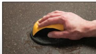
When the mark has been removed you will then need to use the grey abrasive pad to return the surface to the original finish. Cover the same area that has been sanded plus a slightly wider area to blend in.
