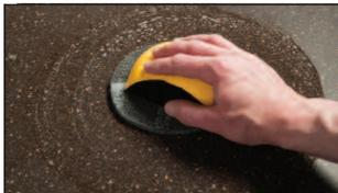
Using the foam sanding block, rub over the affected area in a circular motion. A slight paste will be generated that aids the scouring process and helps to maintain the original level of surface finish.
