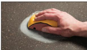
Using small circular movements, work a small area around the affected part of the surface. A small amount of dust will be generated - this will need to be wiped off to check progress.
