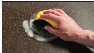
Cover the affected area with a liberal amount of soapy water. Place the grey abrasive pad onto the wet surface.
